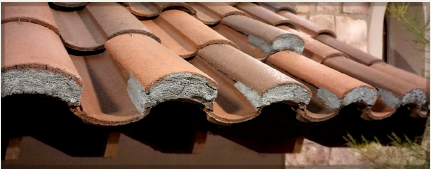
Close-Up of Boosted Eave
